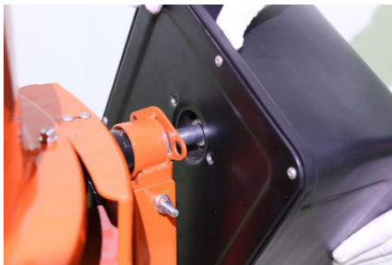
Assemble the motor Fix the motor on bracket with tools
